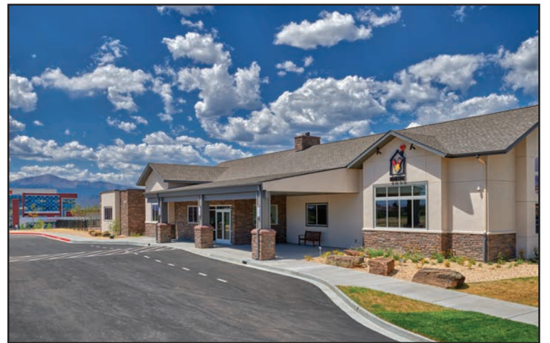
The new Southern Colorado Ronald McDonald House was constructed on the campus of the new Children’s Hospital in Colorado Springs so families could be close to their critically ill child. Family suites in the west-facing areas of the new House also provide incredible views of Pikes Peak.
